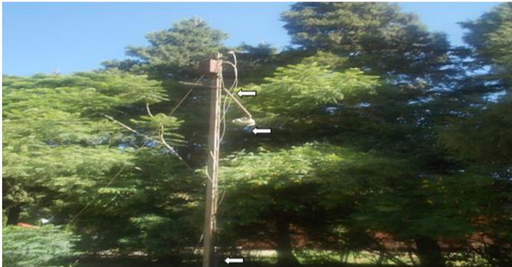
Plate 1.3: Street Lighting in a State of Disrepair in Gweru East. Broken electricity lines indicative of non-functioning street lights with arrows
